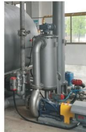
自清洁过滤器 Auto lint cleaning and filter
